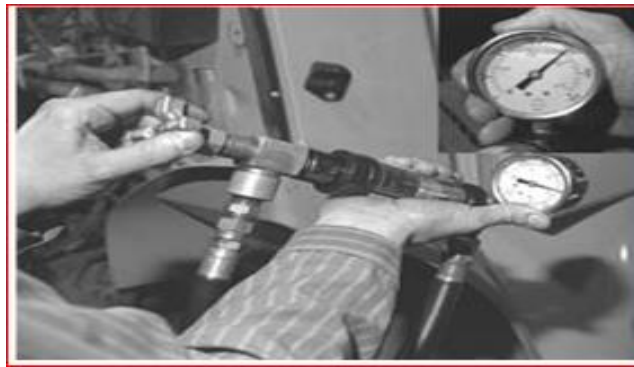
Figure 2:36 Test the pump relief valve and flow control pressures
