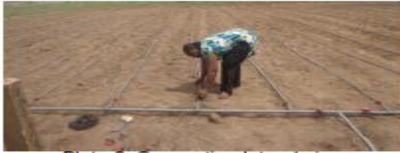
Plate 3: Connecting lateral pipes
